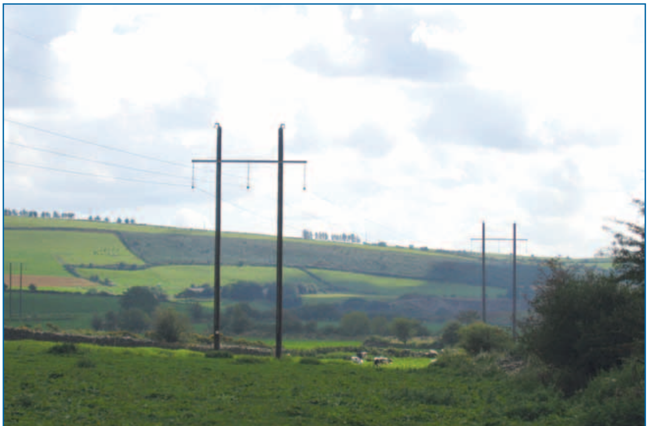
Figure 1.3: Single Circuit 110 kV Overhead Line Design
