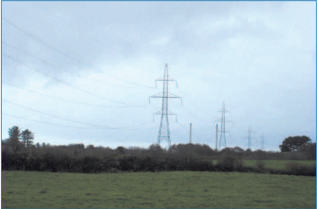
Figure 8.2: An existing 400 kV double circuit line close to Moneypoint generating station in County Clare
